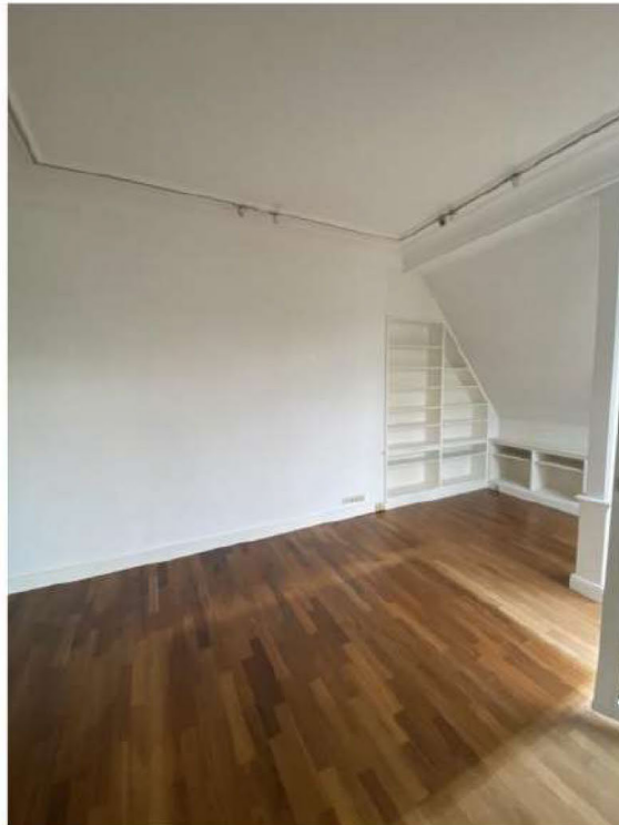
Before the renovation
